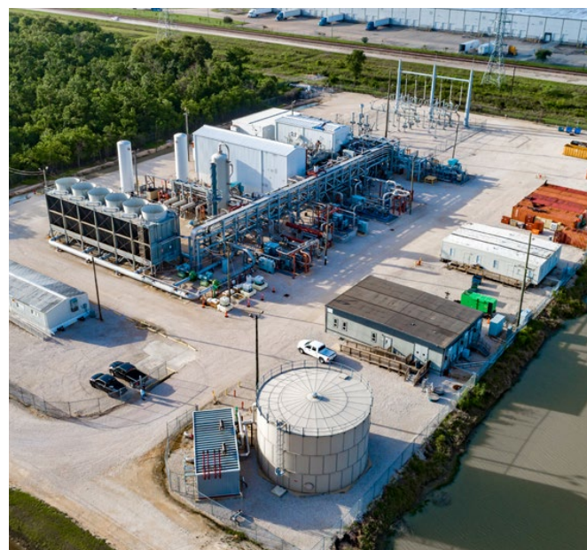
Net Power's La Porte Test Facility
