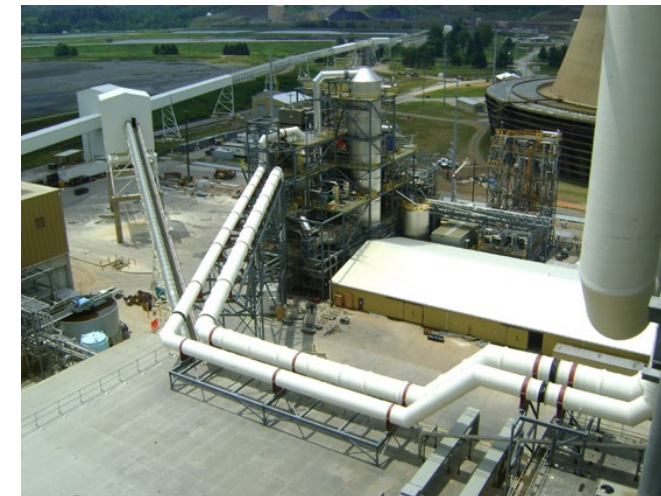
American Electric Power (AEP) Mountaineer Station
