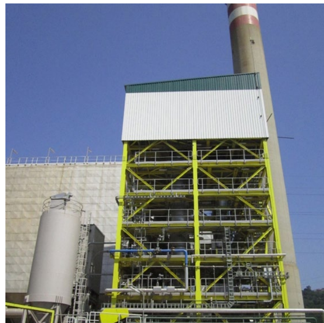
Calcium Looping 1.7 MW demo plant completed in La Pereda, Spain. The pilot plant was commissioned in 2012 with demonstrated capture efficiency of over 90%
